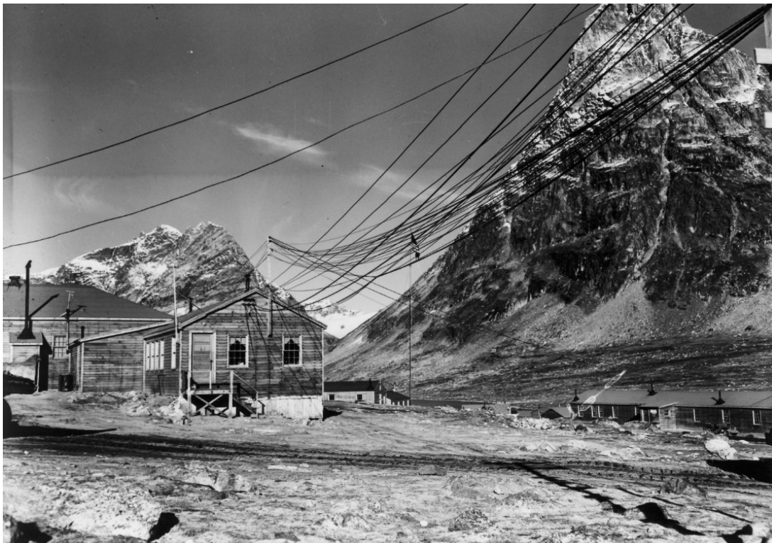
Fig. 20. BE-2's electrical grid and connecting telephone communications. The grid was quite extensive and ran in-between the various buildings on the base. Staff Sgt. Harry M. Baar photo archive 1944-1945, Greenland National Museum and Archives.
