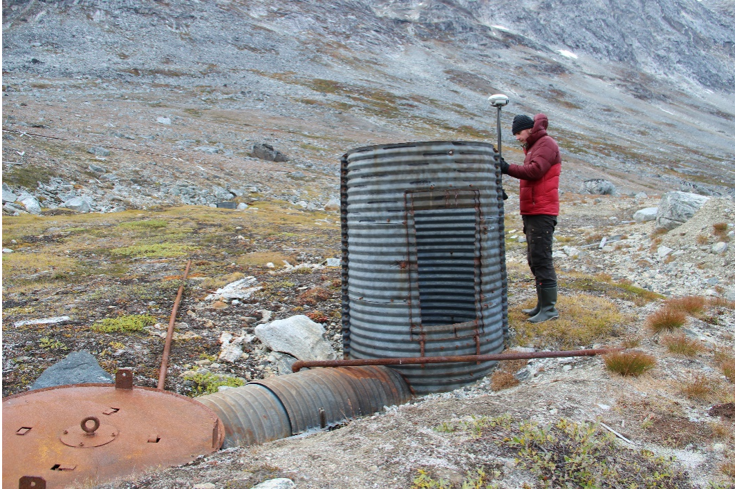
Fig. 16. A corrugated metal housing resting on top of the camp water catchment well at BE-2. At the time of the visit in 2018, water could still be heard to be flowing into and out from the well (photo; H. Lange 2018).
